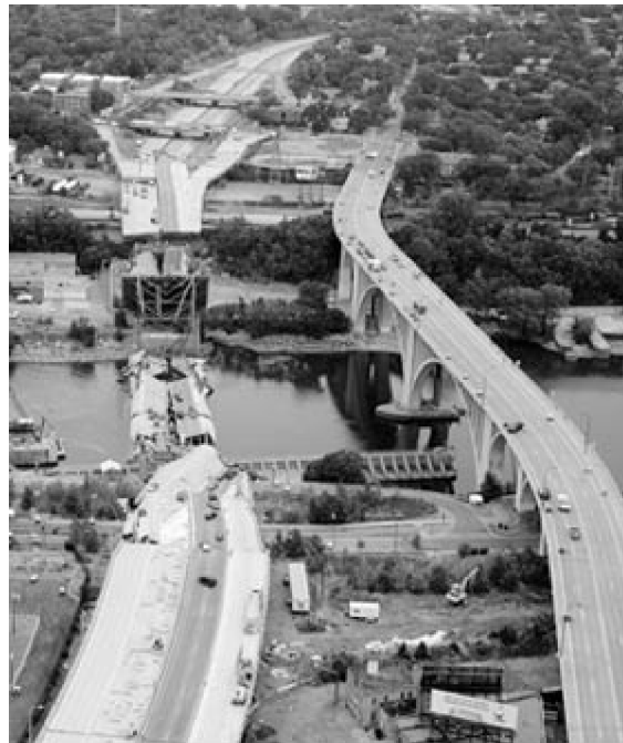
A view of the collapsed Interstate 35W bridge, August 4
